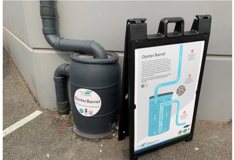
Figure 1. Oyster shell downspout barrel system and information sign at Terminal 102
